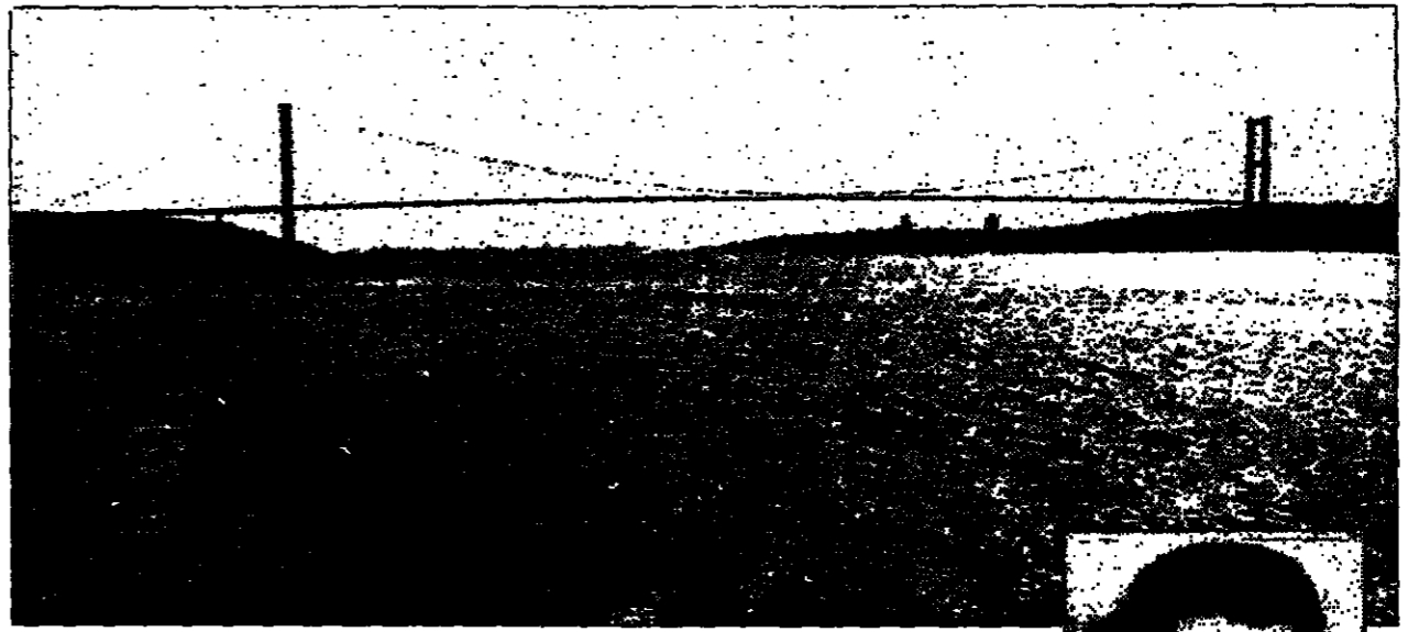
The Bosphorus bridge linking East and West.
